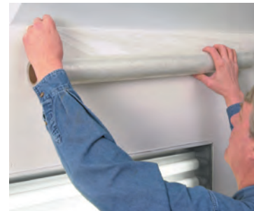
Beginning at one end of the wall, tack down a 2"-3" starter edge at the ceiling break.
